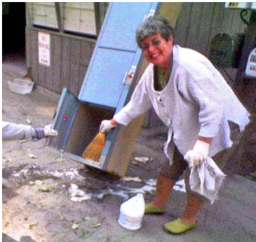
Parcel Locker Rehab
